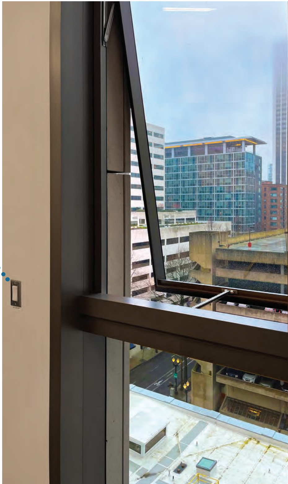
Multnomah County Courthouse
